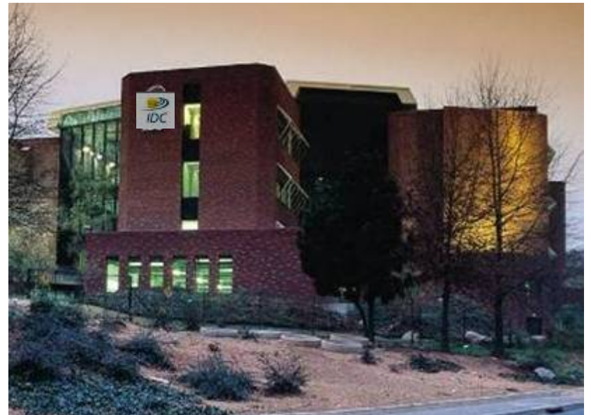
The IDC's Head Office in Sandton (Johannesburg)
